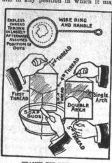
FRAMES FOR THE FILMS. happen to fall. But if the film is bro below this thread it will be pulled up into a circular arch by the tension of the contracting film above.
