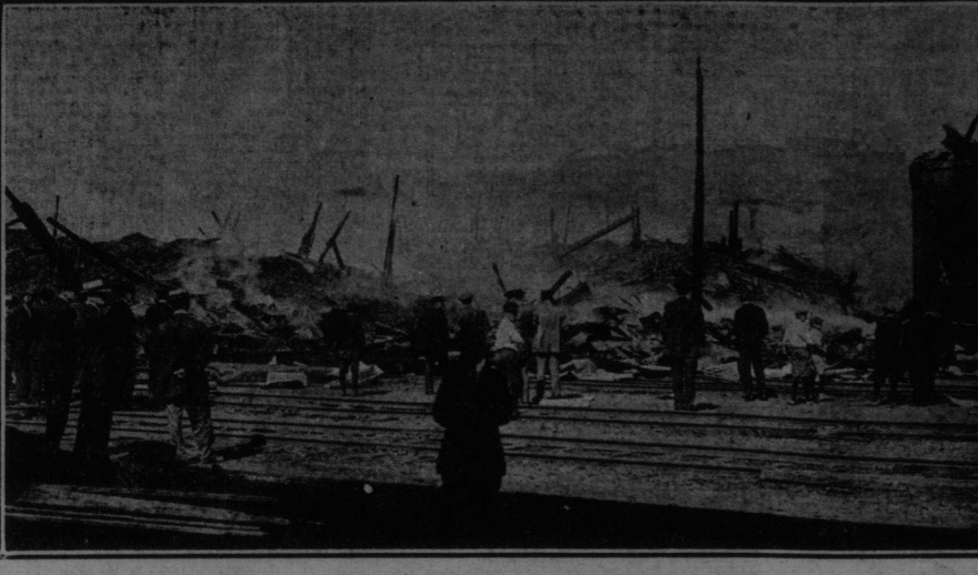
SMOKING RUINS OF I. C. R. GRAIN ELEVATOR, NEAR UNION DEPOT, THAT WAS DESTROYED BY FIRE WEDNESDAY NIGHT—SNAPPED BY THE STANDARD STAFF PHOTOGRAPHER.
