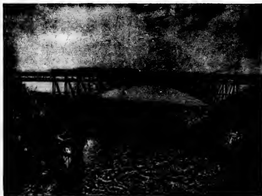
G. T. E. Single Span Steel Bridge over Niagara River.
