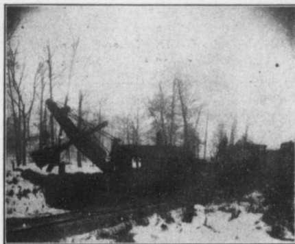
Giant Class E 65-ton Steam Shovel.
