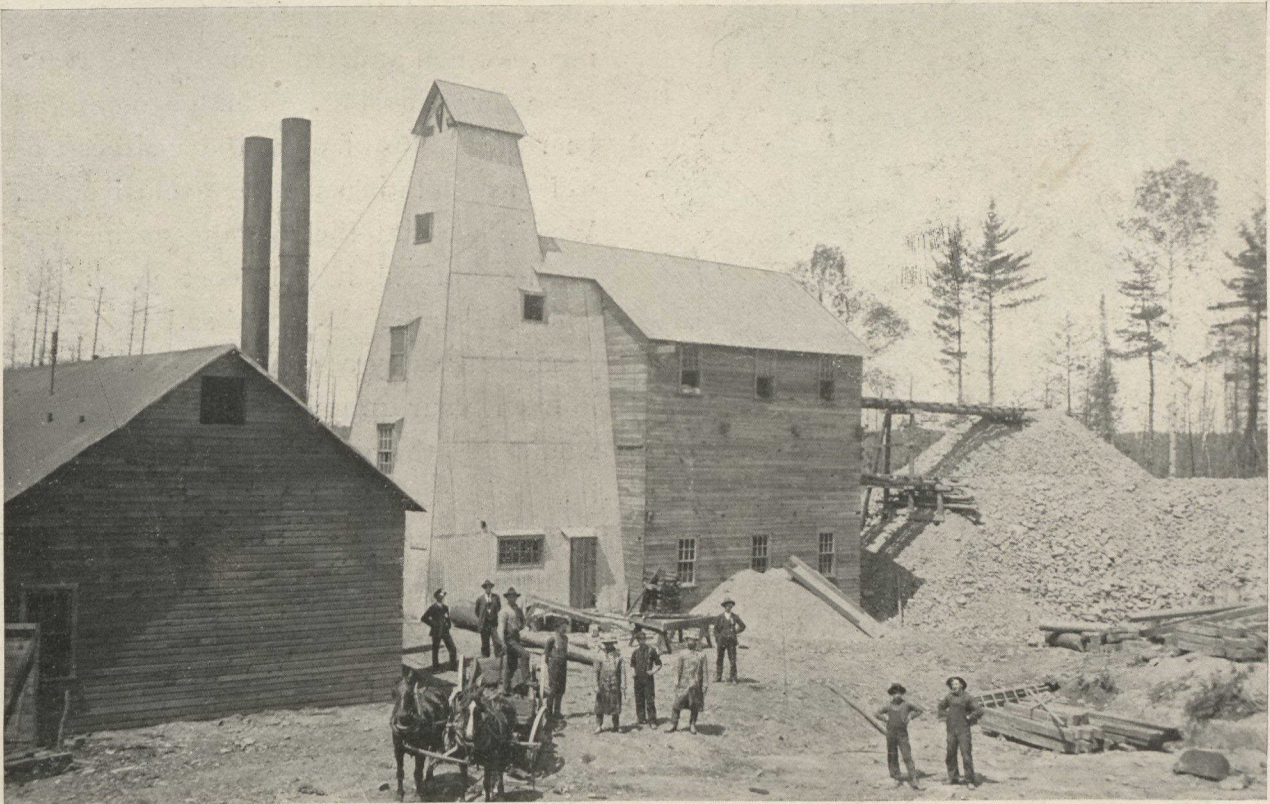
A TYPICAL SHAFT HOUSE.—COBALT.
