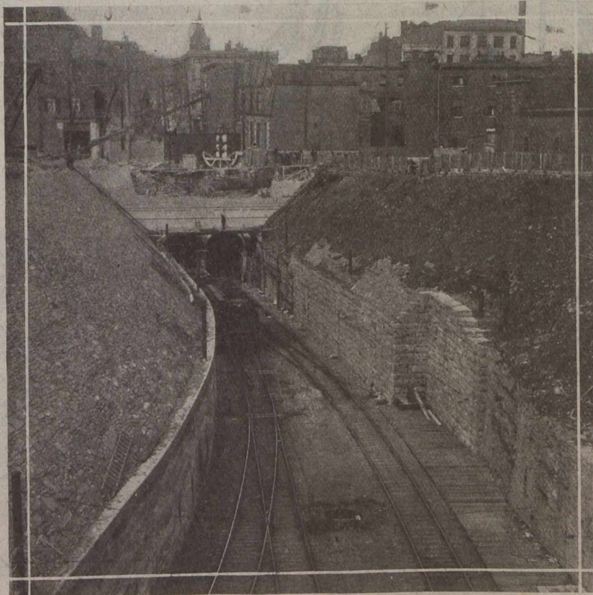
THE MONTREAL PORTAL OF THE C.N.R. TUNNEL
