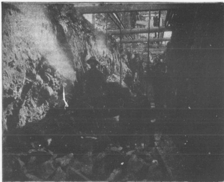
Three out of the ten or our "Ingersoll" steam drills used by Messrs. Laurin and Leitch in excavating rock at St. Louis de Mile End, Quebec. These rock drills are fully described in catalogue No. 81
