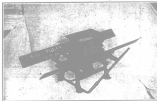
Is the only all-purpose machine on the market. Any size block in length, width or height, as required. Keystones and arch blocks can be made just as quickly as square blocks. plates can be adjusted to make blocks to any angle, as it is built on an adjustable sectional plan. Cornice, mouldings, door and window jambs, lintel and window sills. There can be a block
