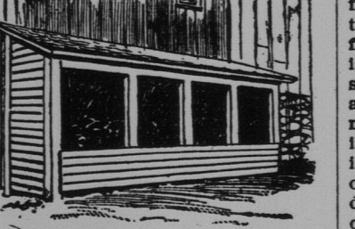
TANK COVERING WITH DOOR UP.
