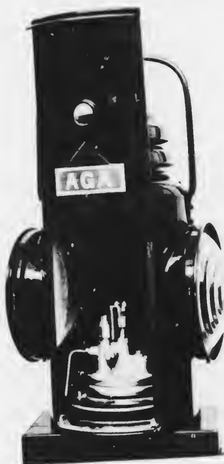
THE AGA SEMAPHORE LAMP WITH FLASHER MOUNTED.
