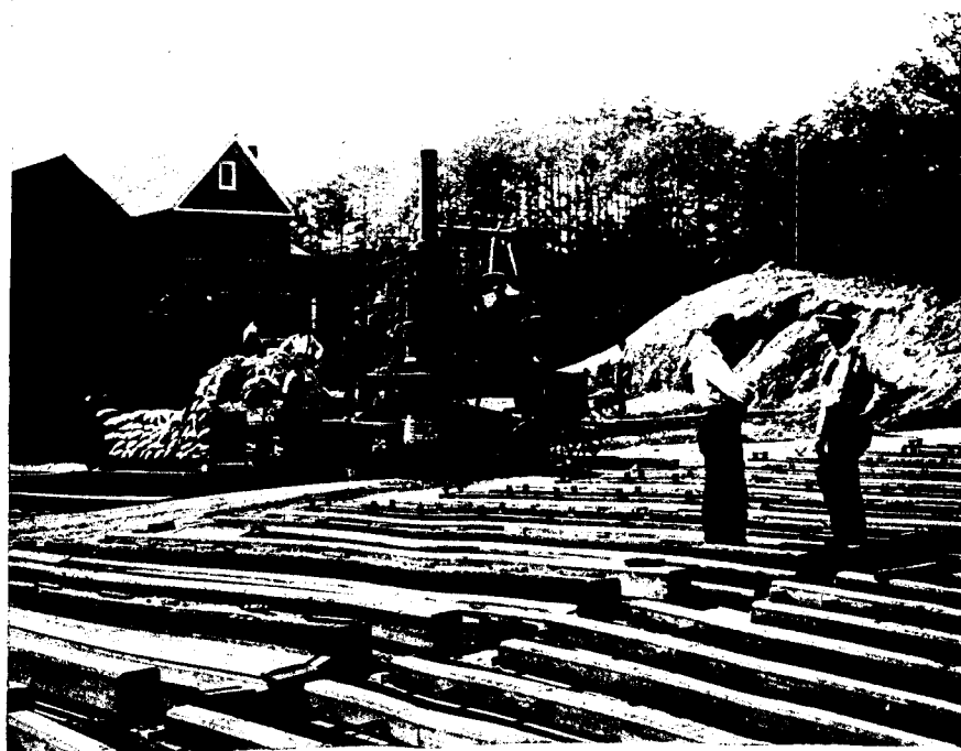
Wettlaufer Heart Shape Mixer making Hydro Electric Poles at plant on Spadina Road.
