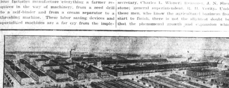
MASSEY-HARRIS COMPANY'S PLANT AT BRANTFORD.
