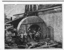
Large Buffalo Steel Plate Fan for mechanical draft is shown in course of erection. We undertake to design and install these fans assuming full responsibility for results.
