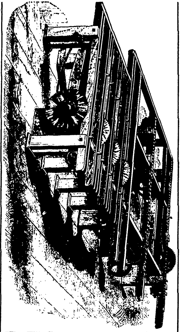
IMPROVED DOUBLE EDGER (THICK & THIN SAW.)
