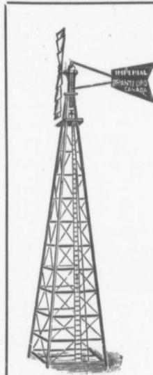
**O**UR TOWERS are girted every five feet apart, and double-braced. This doubly insures against accidents in storms. All Mills are galvanized after completion. This gives increased strength.
