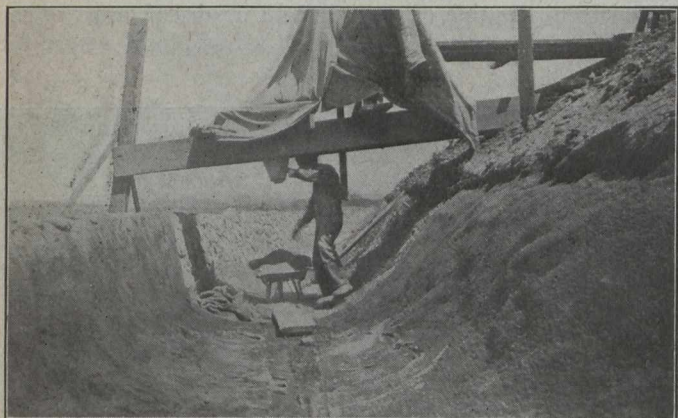
Fig. 5.—Loading Wheelbarrow from Hoppers
