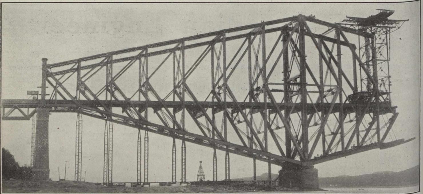
Comparing this view with that shown in *The Canadian Engineer* for December 31, 1914, page 797, indicates this year's progress of erection on the North Shore. The "flying bridge" is also shown in place.
