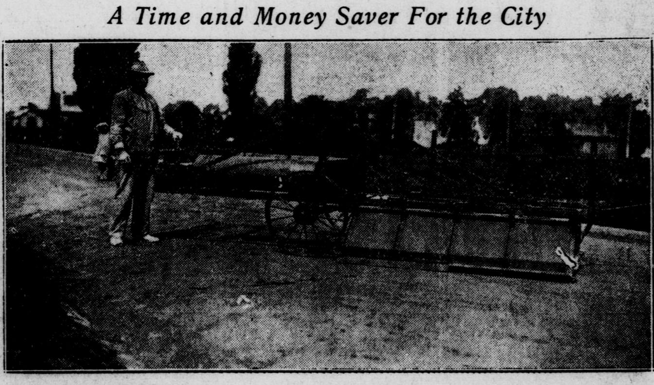
The Free Press Photographer. This is the new oil burner which was recently purchased by the city for use in repairing the pavements. The surface is melted in order that it can be shoveled up, which saves much time over the old method, in which the surface had to be broken up with picks. There are six burners under the hood in the front. The burners are fed from the coal oil tanks seen in the rear. The machine, which was built by the Waterous Company, of Brantford, will be used for the first time next week.
