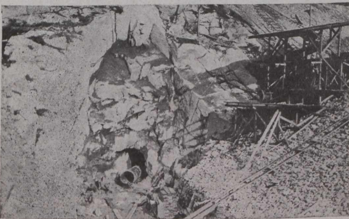
Fig. 5.—Foundation for Water Tower—4-ft. Pipe in Entrance of Tunnel. Note Solid Rock Foundation.
