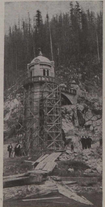
Fig. 7.—Water Tower, Front View.
