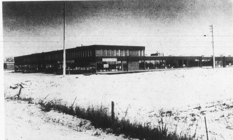
One of three new commercial outlet along Dundas, this plaza is located opposite Dixie Arena.
