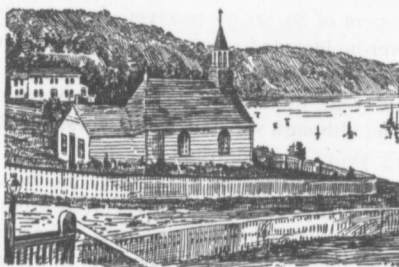
THE JESUIT CHAPEL IN TADOUSSAC. BUILT 1647. THE SECOND OLDEST CHURCH IN AMERICA.
