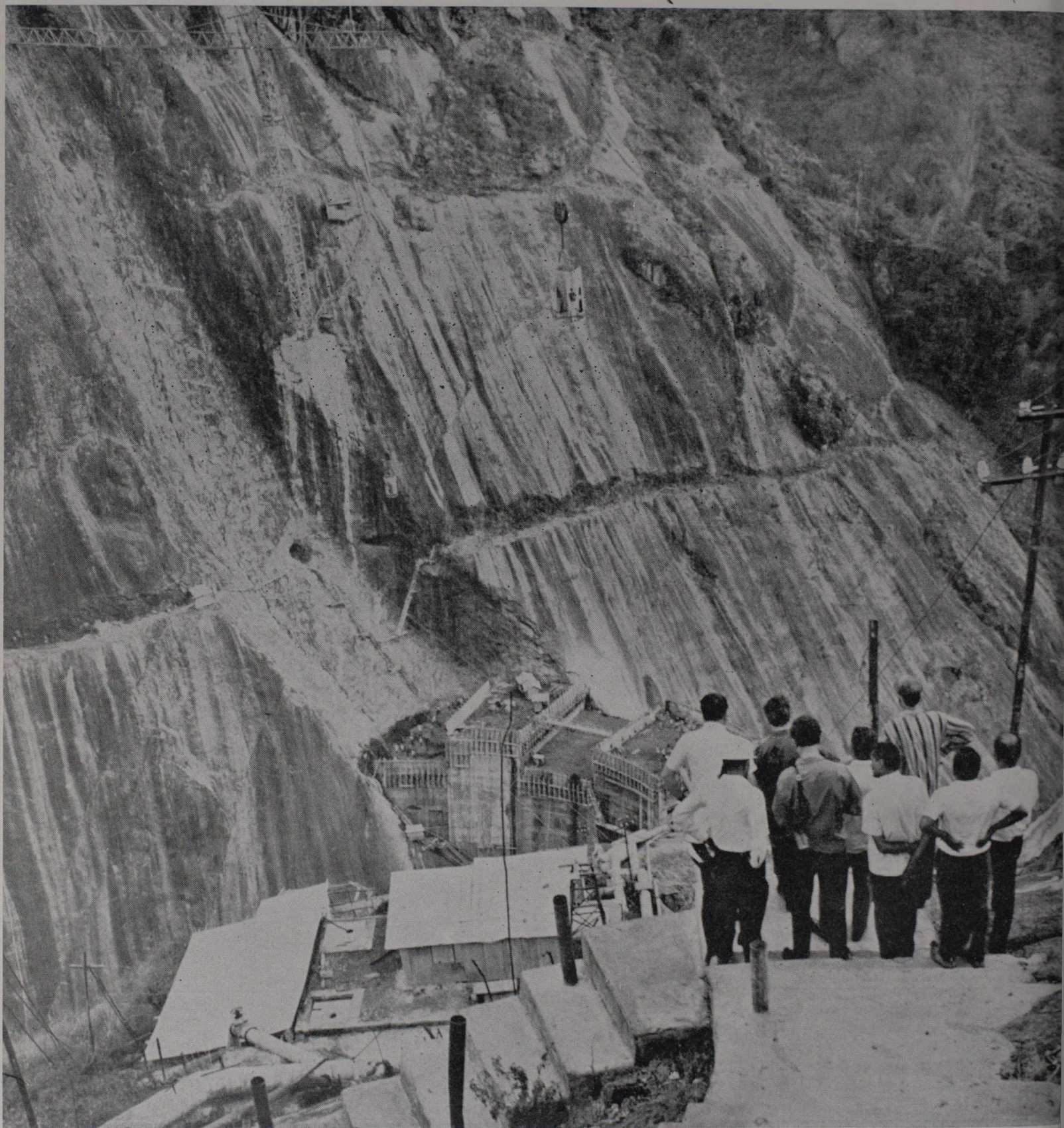
Mr. Gerin-Lajoie viewing the Idikki Arch Dam. Located on the western side of the Nilgiris, in Kerala, the project is changing the face of the Periyar Valley. With an installed capacity of 780MW (for peaking), Idikki will be the biggest hydro-electric scheme in South India. The 560 feet high arch dam will be the first arch dam in India and the highest in Asia, over three times the height of Niagara Falls. Besides cheap power, the project will irrigate 150,000 acres via canals downstream.
