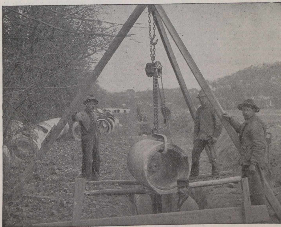
A Triplex Block hung from a temporary rigging and used for laying pipe.
