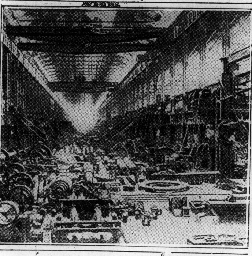
MACHINE SHOP NO. 4 AND CRANES WHICH SAVED GUNS. While the flames were at their height in the great fire which destroyed the big machine shop of the Bethlehem Steel Company, at South Bethlehem, Pa., the electric travelling cranes on the main floor were operated to remove as many of the eight hundred guns in the building as possible.
