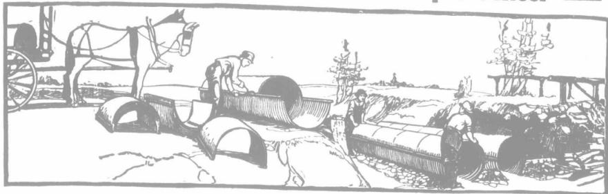
**EASILY-LAID** Pedlar Corrugated Culvert made in non-rusting 'Toncan Metal' is handled "right at the job" and placed by a couple of men in a few hours' time. It makes a frost-proof and freshet-proof culvert—outclassing wood, masonry, concrete or brick. Strong enough to hold up a traction engine on the bare ground. Get our book. See Pedlar Culvert's uses for farms and roads. We send you a free sample, too. This is the best, strongest, deepest corrugated culvert ever made. Write for book.
