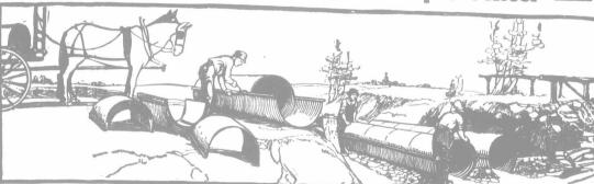
made in non-rusting 'Toncan Metal' is handled "right at the job" and placed by couple of men in a few hours' time. It makes a frost-proof and freshet-proof culvert proof freshet-proof culvert proof freshet-proof culvert proof and freshet-proof culvert proof freshet-proof freshet-proof culvert proof freshet-proof freshet-proof culvert proof freshet-proof a couple of men in a few hours' time. It makes a frost-
