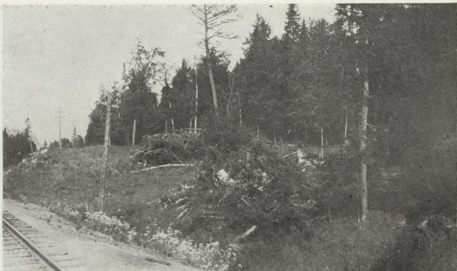
Railway right-of-way in process of clearing. Note large piles of inflammable debris ready for burning. A clean right-of-way is an essential factor in railway fire prevention, but its beneficial effects are largely neutralized if the immediately adjacent lands constitute a fire-trap, through the presence of logging slash and other highly inflammable debris. The safe disposal of logging and other slash in proximity to railway lines should be strictly enforced, in the public interest and as a matter of fair play to the railways.
