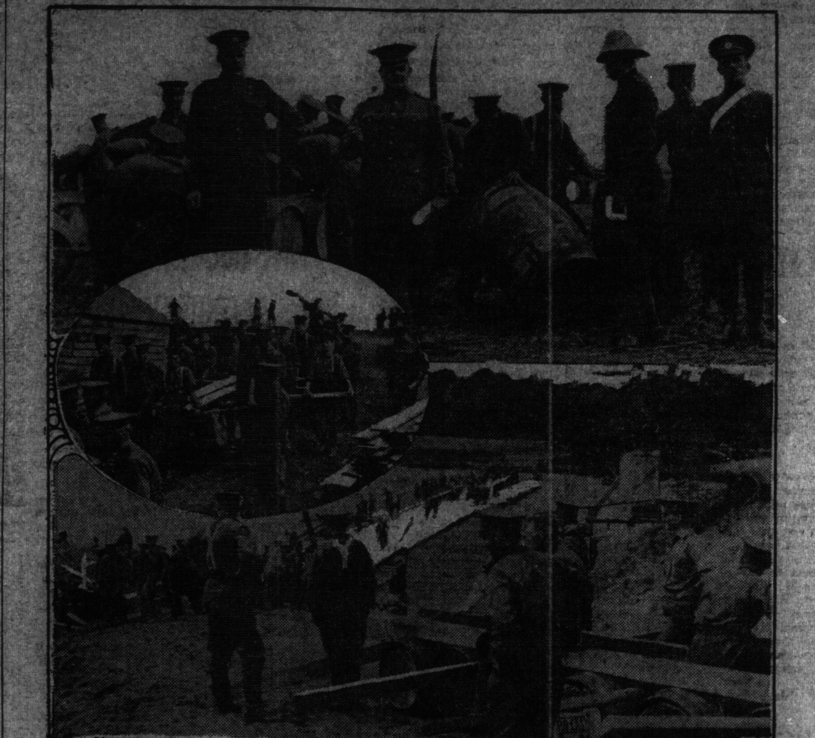
The top picture shows the collecting and lashing together of the barrels, Major Lindsay being the central figure in the picture; in the inset the engineers are shown carrying the sections down to the water, and the lower picture shows the bridge nearly completed.—Photos by courtesy of the Canadian Northern Railway.
