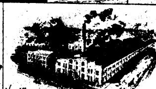
NEW FACTORY BUILT IN 1895 SINCE THEN THE FOLLOWING EXTENSIONS HAVE BEEN MADE MACHINE SHOP LENGTHENED 140 FT NOW 440 x 120 WELD SHOP 100 FT NOW 220 x 80 BUILDING SHOP 100 FT NOW 100 x 40 BLACK SMITH SHOP 40 FT NOW 100 x 40 IN EQUIPMENT.
