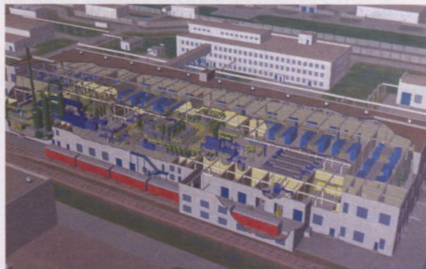
Production Building: Russian Chemical Weapons Destruction Complex
