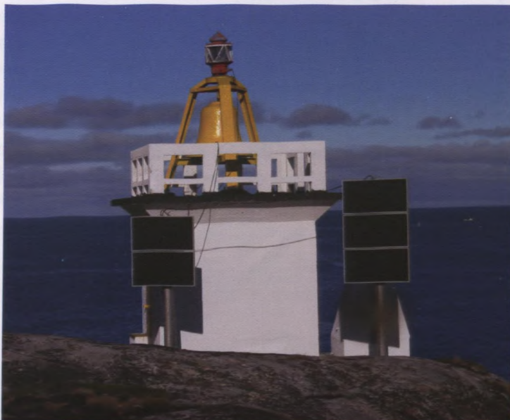
Solar cell panels provide a sustainable alternative power source for lighthouses formerly powered by highly radioactive material
