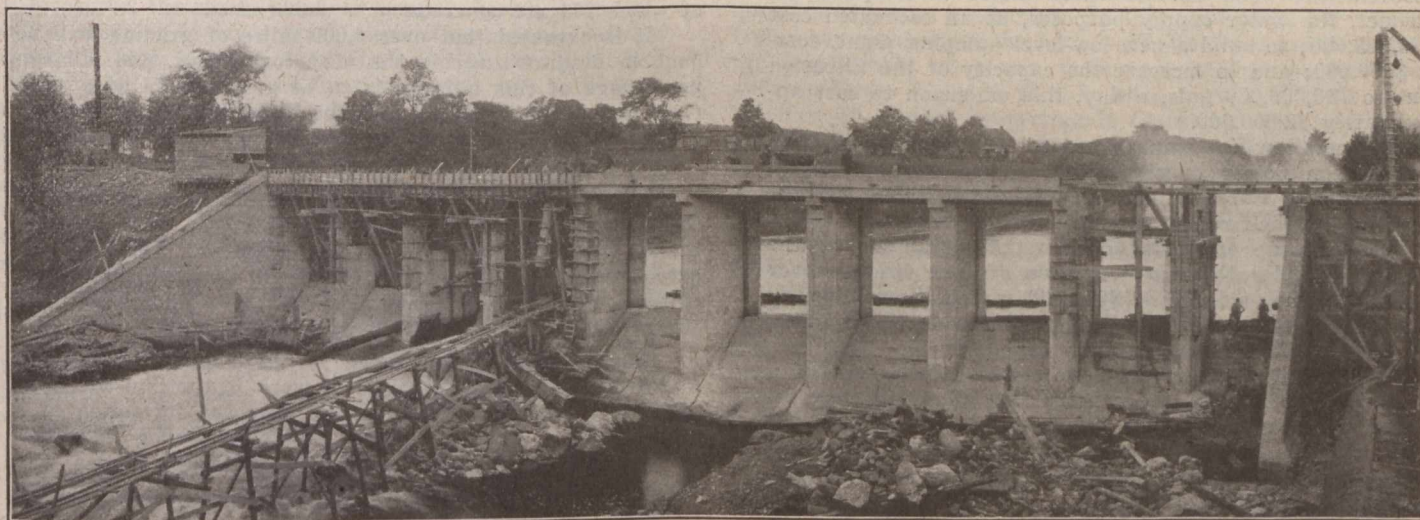
FIG. 7—DAM UNDER CONSTRUCTION—PART OF MIXING PLANT AT EXTREME LEFT—TRETTLE TO POWER HOUSE IN LEFT FOREGROUND
