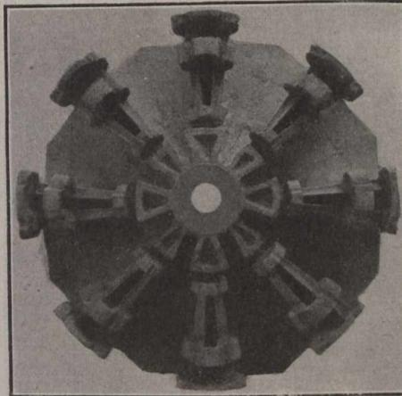
Fig. 5.—Centre Casting of New C.P.R. Snow Plow.
