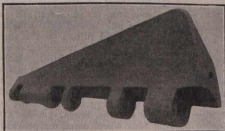
Fig. 8.—Cutter Blade of New C.P.R. Snow Plow.
