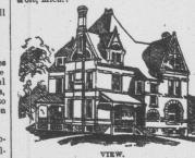
mings, slate roof; principal apartments finished with hard wood, oil finish, inside blinds, etc. Height of stories—first, 10 feet 6 inches; second, 10 feet. Cellar, 6 feet 6 inches. First
