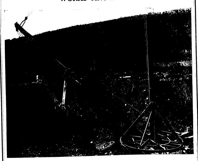
The Bishop Steam Shovel Derrick Attachment adds the service of a Steam Shovel to your Derrickand at a fraction of the usual cost for complete equipment.
