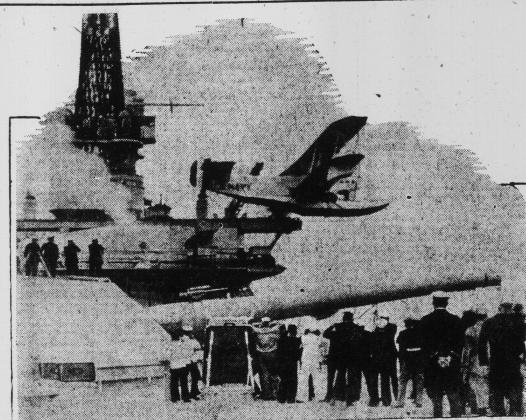
"HISTORY in the making" may be the term applied to the shooting of a 5,100-pound amphibian plane from the top of the turret of the U. S. S. "West Virginia" in Los Angeles harbor. It never had been done before. A charge of powder equivalent to that used in an eight-inch shell was exploded. Lieut. D. S. Fahrney piloted the plane in the experimental take-off.
