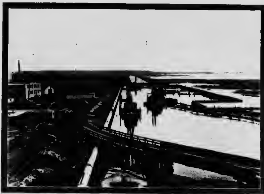
HARBOR COMMISSION HYDRAULIC DREDGES DRIVING THE NORTH SLIP THROUGH THE NORTH PART OF THE INDUSTRIAL DISTRICT.
