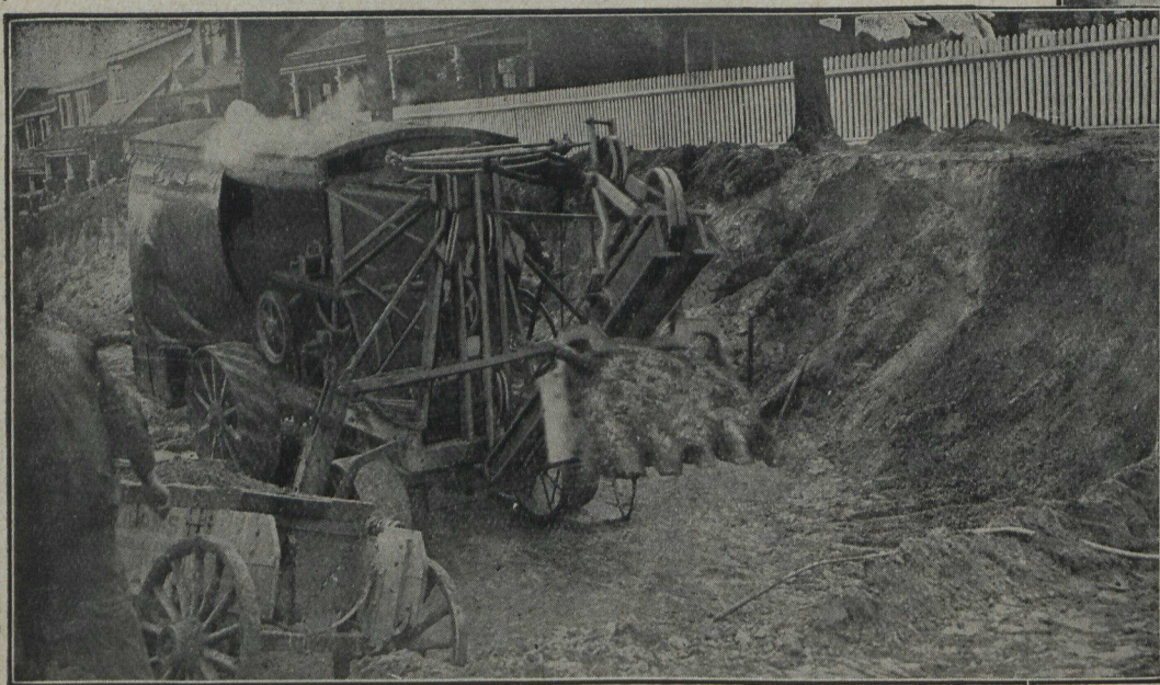
Keeping the dump wagons moving in a Toronto grading job with the Keystone.
