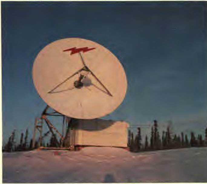
This earth station at Inuvik in the Northwest Territories is one of 100 in the national network of Telesat Canada, an enterprise owned jointly by the federal government and Canadian telecommunications carriers.
