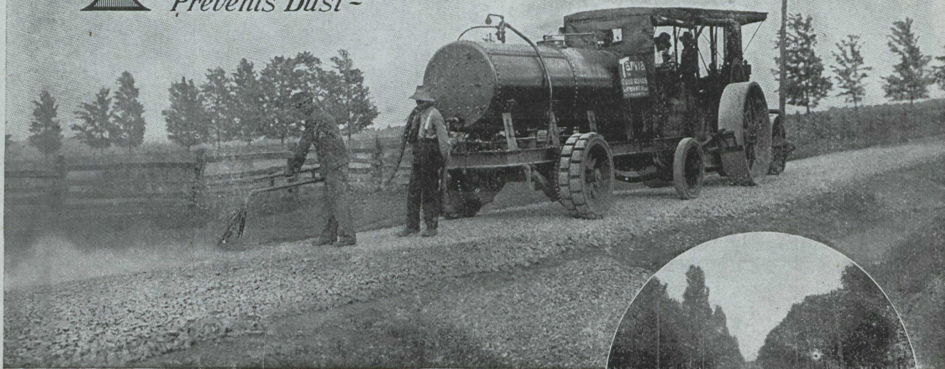
The above illustration shows the spraying of hot "Tarvia-X." The view in the circle is the finished road. It is durable and dustless.
