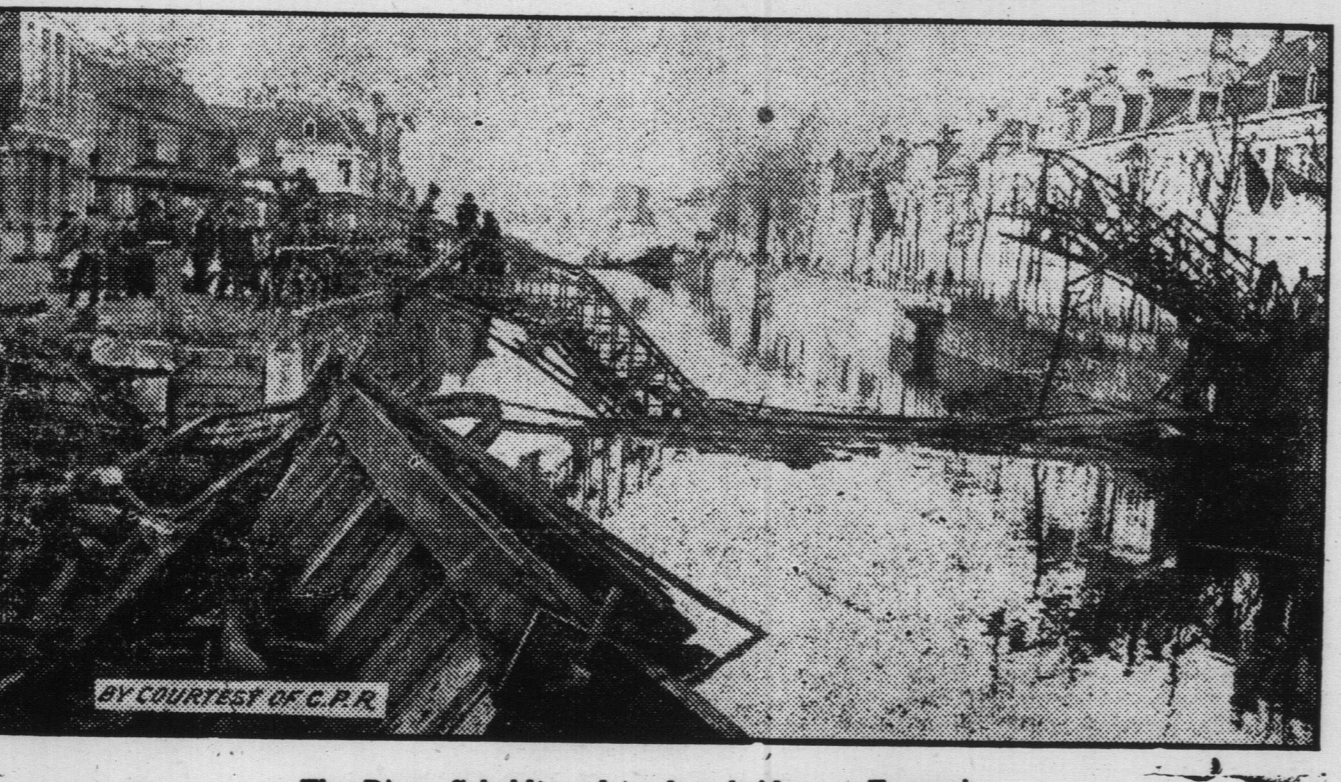
The River Scheldt and broken bridge at Tournai.
