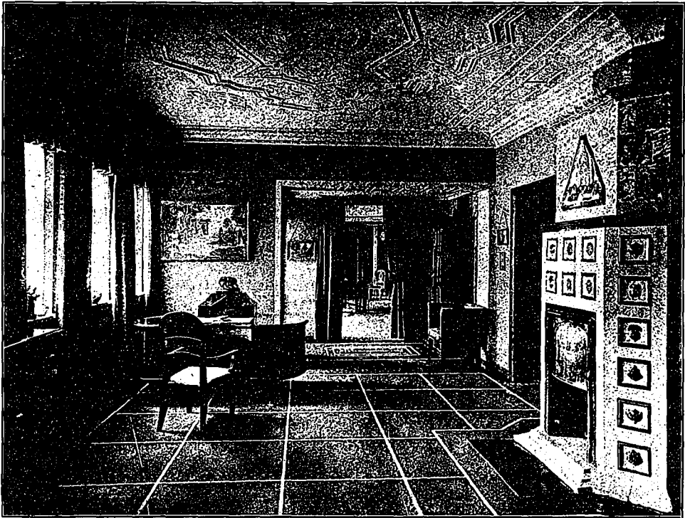
SHOWING DOLOMENT FLOORING AS USED IN BUSINESS OFFICE.
