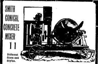
Mixes in Batches. Discharges by Tilting while Running. Mounted on Skids or Trucks. Catalogue on Application.
