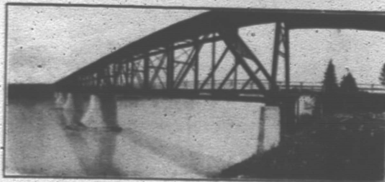
Steel Bridge on Concrete Piers over the Saskatchewan River, at Fort Saskatchewan, 17 miles from Edmonton. One of the five bridges by which the Canadian Northern crosses the North and South Saskatchewan Rivers.
