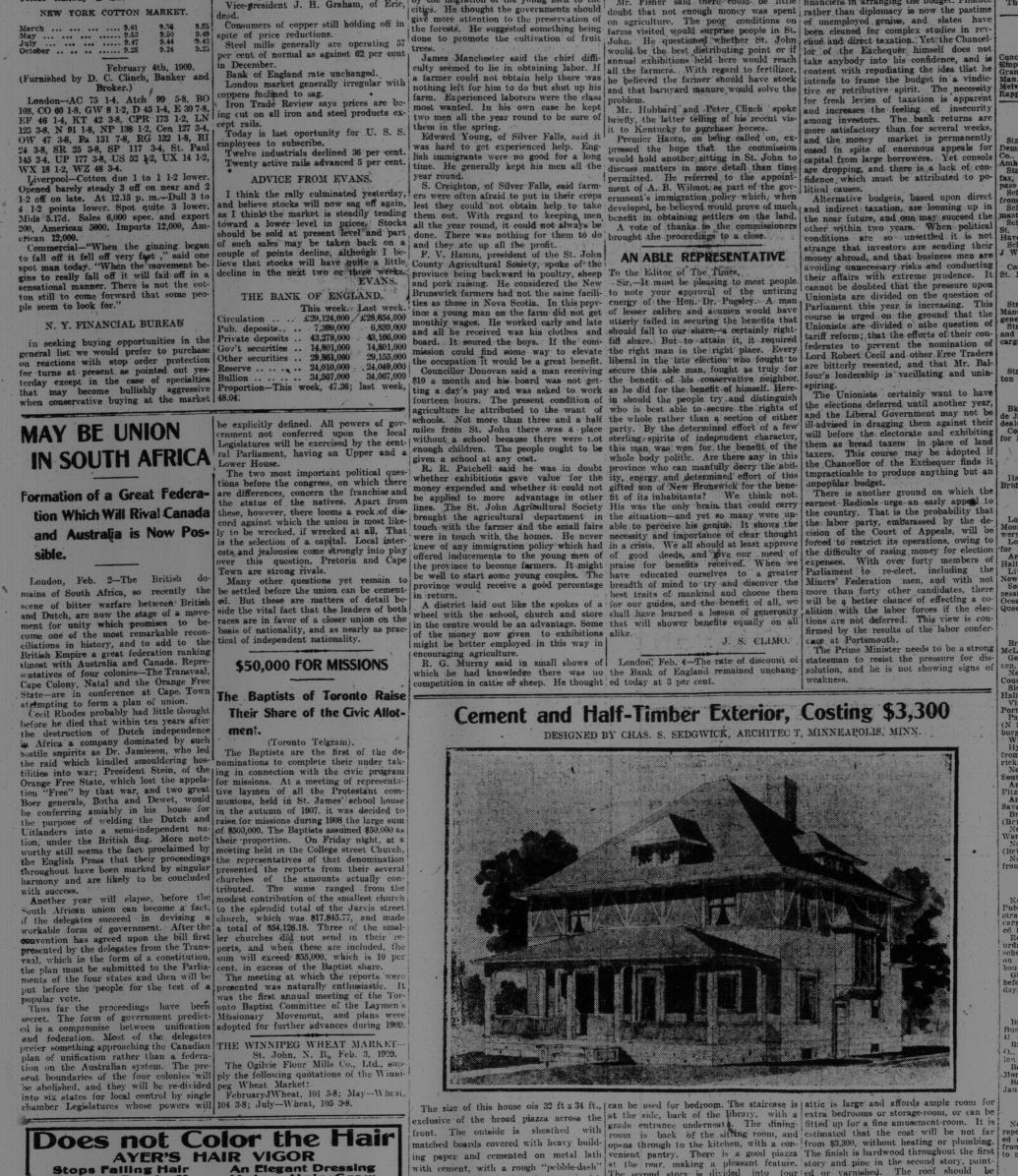
The size of this house ois 32 ft x 34 ft., exclusive of the broad piazza across the front. The outside is sheathed with matched boards covered with heavy build-ing paper and cemented on metal lath with cement, with a rough "pebble-dash" finish. The entrance is in the centre, with a liberal sitting-room on the left-hand side, that
