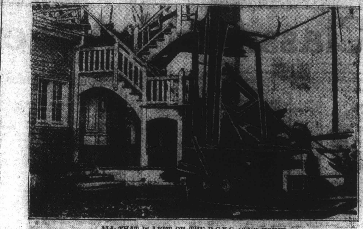
ALL THAT IS LEFT OF THE R.C.Y.C. CLUB HOUSE. The Photo shows here the standing shell of the R.C.Y.C. building, as it looked after the fire was quenched. The main building is so completely gutted that nothing of it is worth saving. To the right may be noticed the tall flag staff, which is charred and blackened on the side next to the fire. The picture gives a glimpse of the attic through which the fire swept with great speed.
