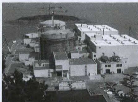
A view of Qinshan III Unit 2 and Unit 1 (background)
