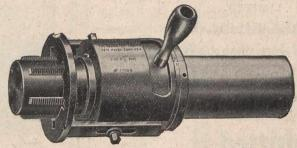
After a hole is tapped the desired depth, the Chasers automatically recede, allowing the tap to be withdrawn
