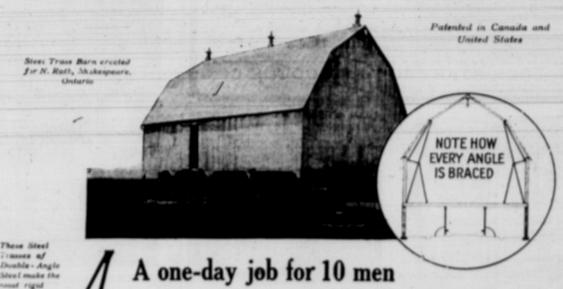
Think of it! Ten men put up the frame of this an-foot barn—put it up ready for the covering of galvanized corrugated bran in one day. The barn left our factory ready to go. uc. not a timber in the whole barn that could not be handled by one man. The trusses were put together at the factory, ready to hold into place.
