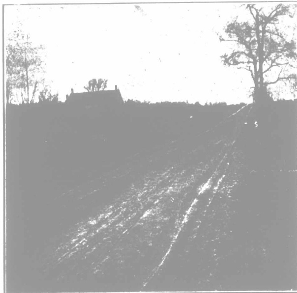
Graded and Maintained with the Split-log Drag.
